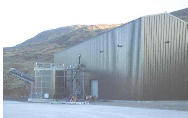
Sludge de-watering building
