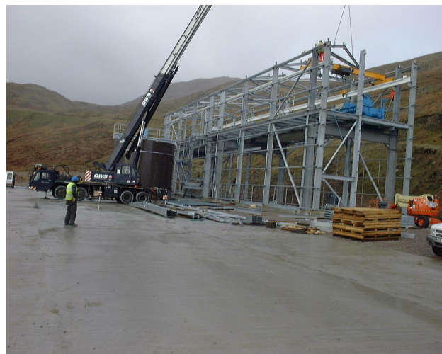
Installation of 2.1m 2 Filter Press—Foster Yeoman, UK
